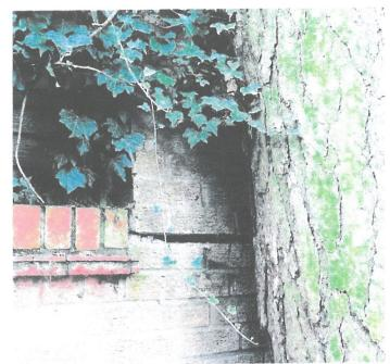
scheme that was proposed by Ward Cole did not address the fact that the trees at the time were in contact with the wall and specifically the parapets that were fractured horizontally by the direct contact of the trees were not reinforced. Therefore, inevitably, further damage has occurred to the wall leaving the parapet, where trees are in contact with the in dangerous wall. enclose condition. 1 photograph of the parapet location and note that the
